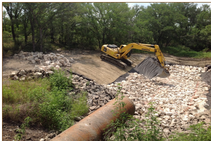
Site # 14 repair of the plunge basin
