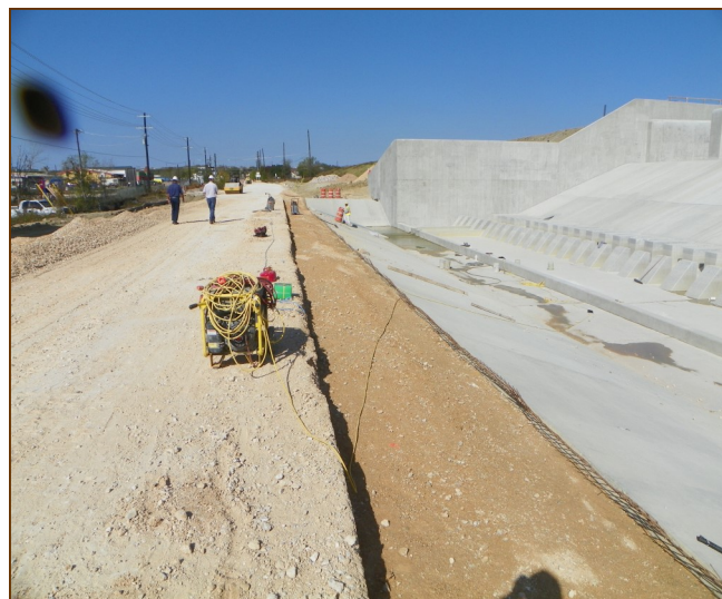
Below site 6 and the construction of Goforth road
