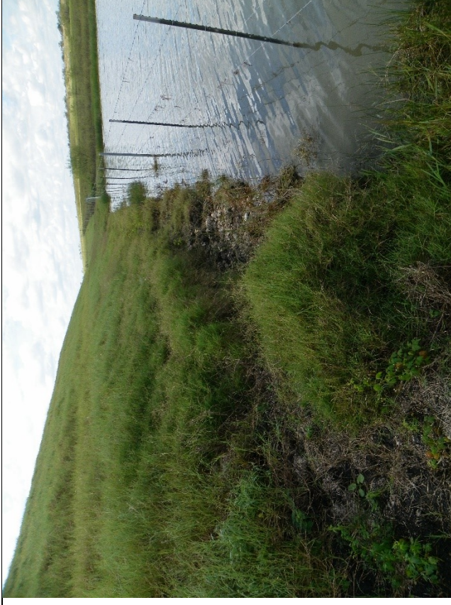
Figure 8. Site 11 -- Looking Left to Right, The Wave Berm Repair Area Along Upstream Slope of Embankment with Fencing that is to be Removed and Reconstructed
