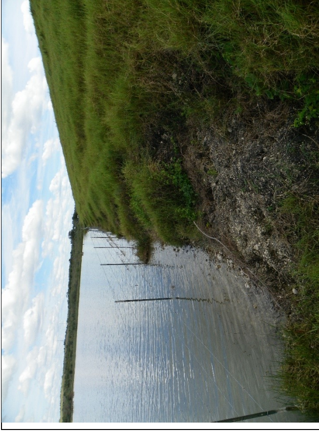
Figure 9. Site 11 -- Looking Right to Left, The Wave Berm Repair Area Along Upstream Slope of Embankment with Fencing that is to be Removed and Reconstructed
