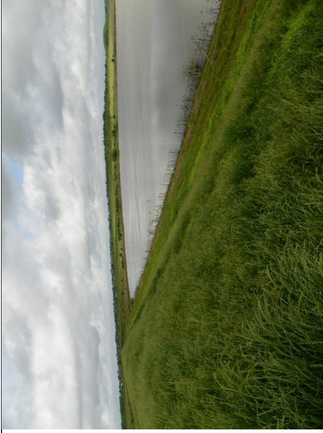
Figure 8. Site 16 – Upstream Slope of Embankment from Top of Embankment Looking Left to Right at Wave Berm Repair Area and Fencing to be Removed and Reconstructed.
