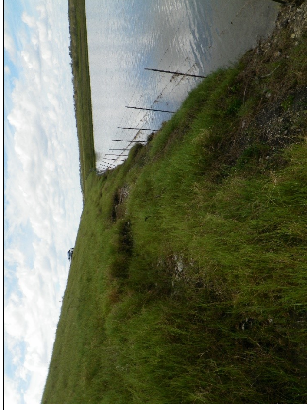
Figure 12. Site 11 -- Looking Left to Right, The Wave Berm Repair Area Along Upstream Slope of Embankment with Fencing that is to be Removed and Reconstructed
