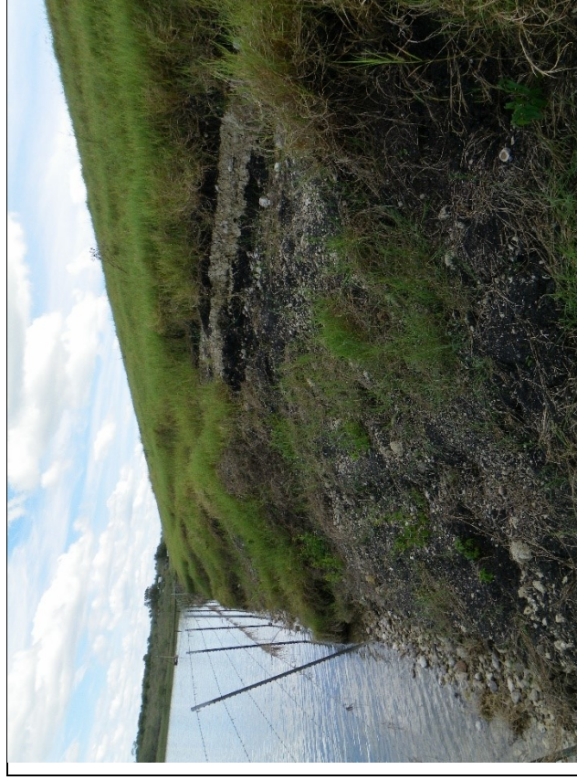
Figure 11. Site 11 -- Looking Right to Left, The Wave Berm Repair Area Along Upstream Slope of Embankment with Fencing that is to be Removed and Reconstructed
