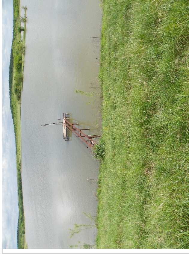
Figure 5. Site 11 – Catwalk from Upstream Slope of Embankment to Principal Spillway Tower That is to be Removed and Salvaged
