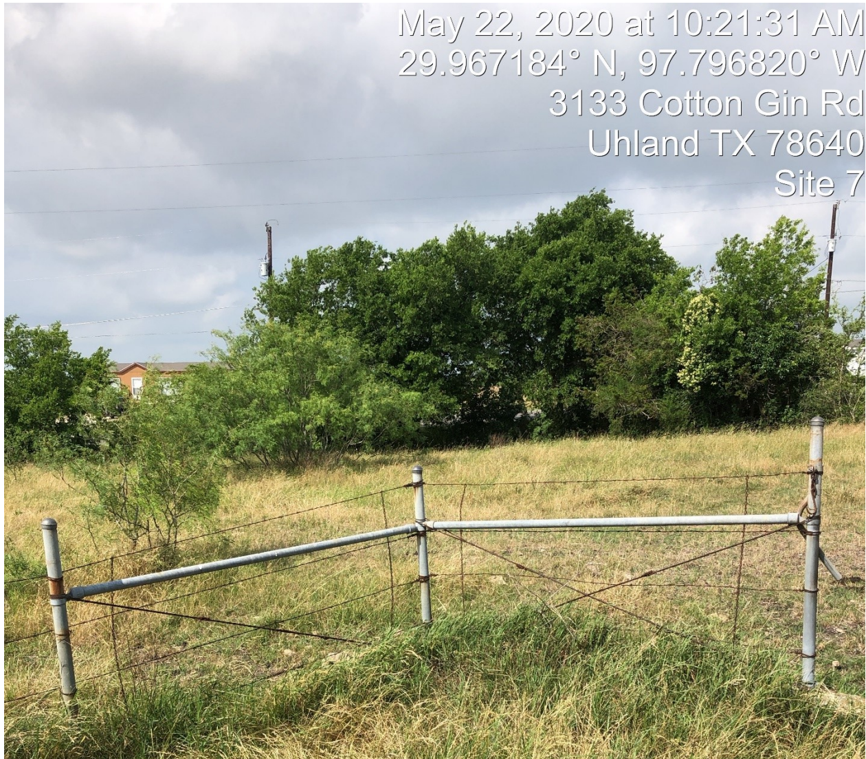
Figure 1. A typical existing corner. Note the cable reinforcements.
