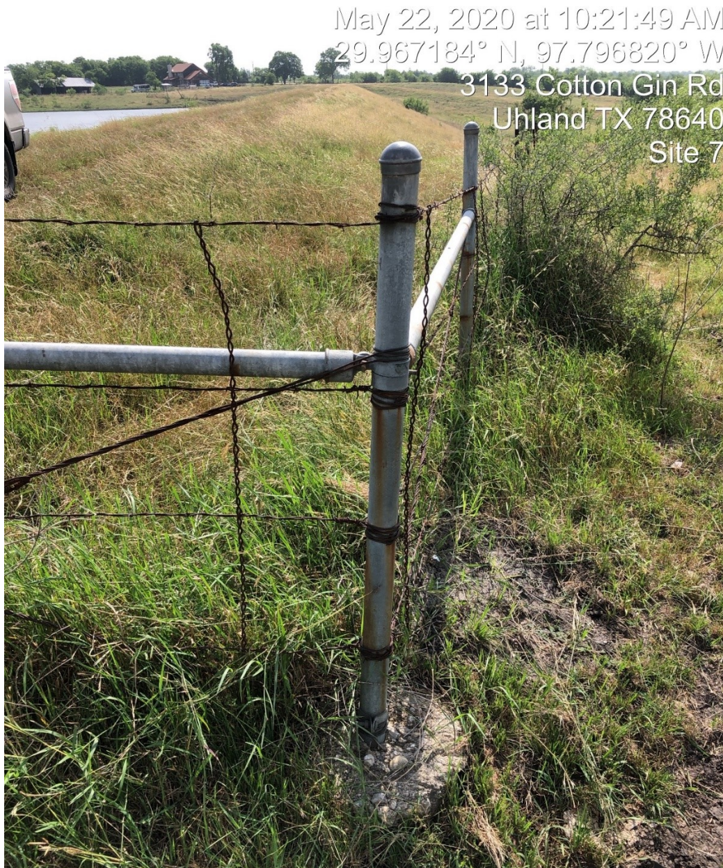
Figure 3. Note that crossbars are joined with bolt and nut.
