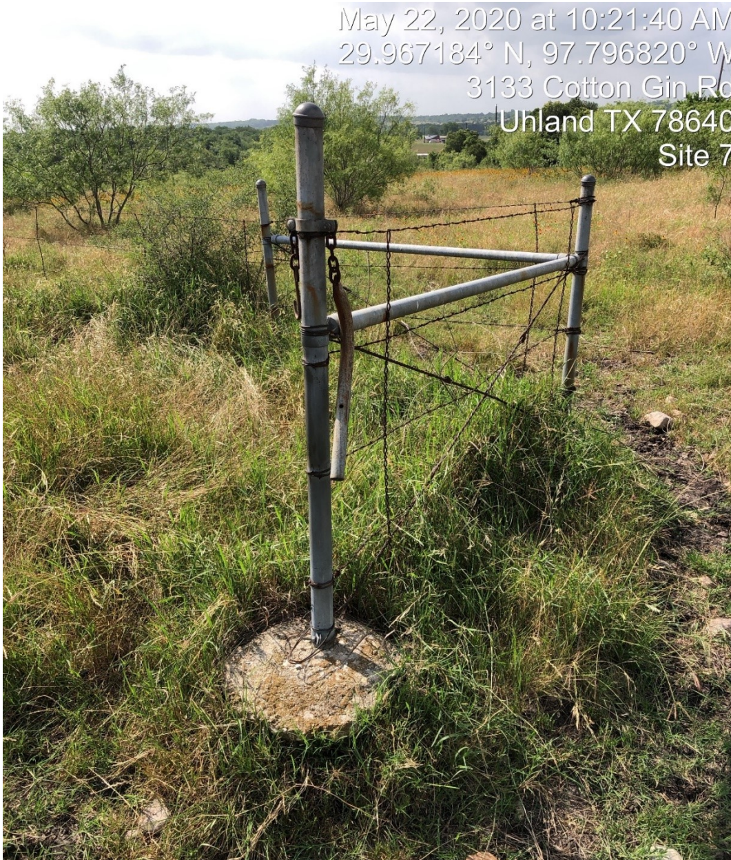
Figure 2. An example of one of the concreted aluminum posts. PCCD Staff counted 39 such posts on a recent site visit. Most corners have three concretes posts. Concrete diameter was observed to be generally 12-18 inches in diameter. Depth of concrete is unknown.
