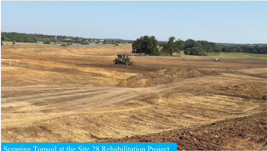
Scraping Topsoil at the Site 28 Rehabilitation Project
