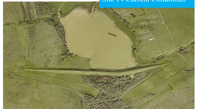
Site 14 Current Conditions
