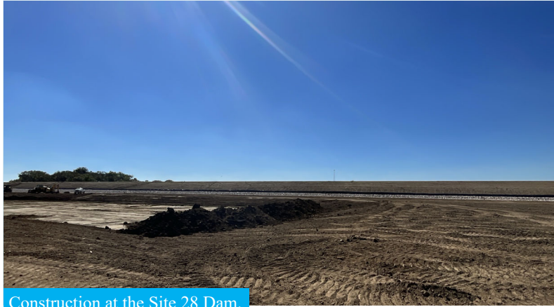
Construction at the Site 28 Dam.
