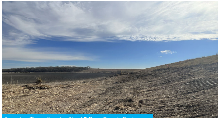
Scraping Topsoil at the Site 17 Dam Repair Project.
